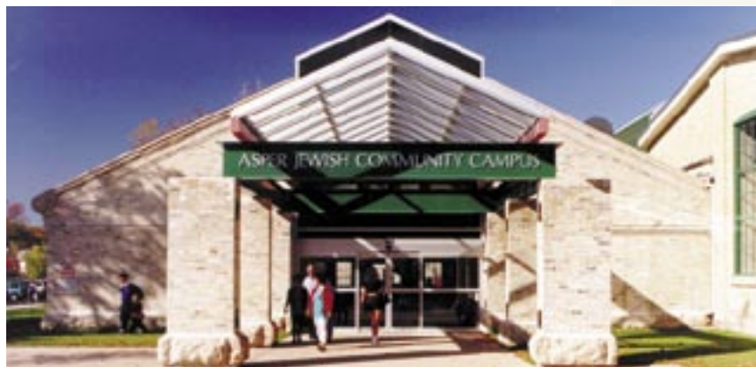
Asper Jewish Community Campus Main Entrance
